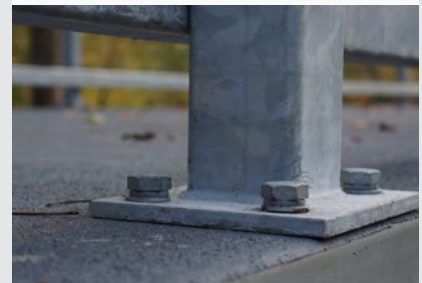
Rail post connections
