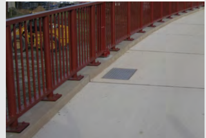
Access openings for utilities
