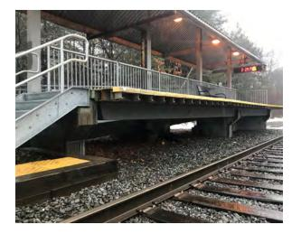
FiberSPAN-R installation replaced existing materials, meeting the specifications and feature requirements outlined by the MBTA. The result is a rail platform deck that performs much better under the harsh environmental and chemical conditions found in the northeast US.
