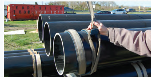
Lift-It® Sling Double Wrapped Around SUPERPILE®
