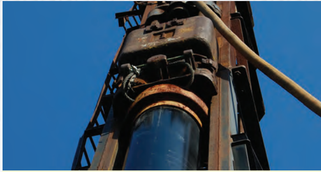
Vulcan 01 Impact Hammer Driving 16" Diameter SUPERPILE®
