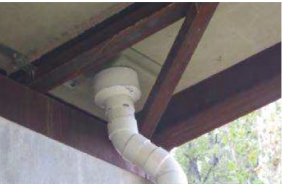
Scupper - Bottom View
