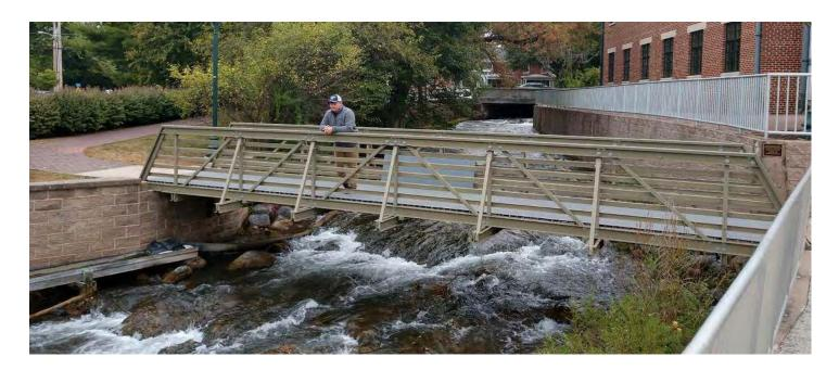
Creative Composites Group designs and manufactures fiberglass-reinforced polymer access structures, such as bridges, boardwalks, walkways and planking. Our product line is prefabricated for quick and simple installation, and is made using corrosion-resistant materials that guarantee years of problem-free use. Our access structures are high-strength while being lightweight, featuring a higher tensile strength than structural steel while weighing 80% less.
