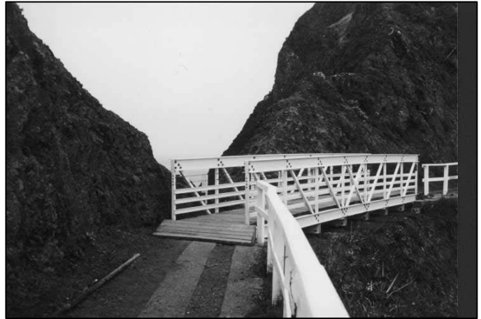
Bridges are easily installed in hard-to-access areas.
