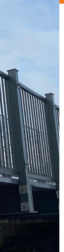
When the Oakville Department of Public Works widened the Speers Road Bridge to five lanes with separated bike lanes, an FRP cantilever sidewalk was an important inclusion. At 94 ft by 6 ft, the sidewalk structure minimized weight by using FRP pultruded elements for channel floor beams supporting the longitudinal decking planks and FRP picket railing on the outboard edge of the sidewalk.
