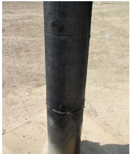
Photo of burnt pole identifiable by the black char
