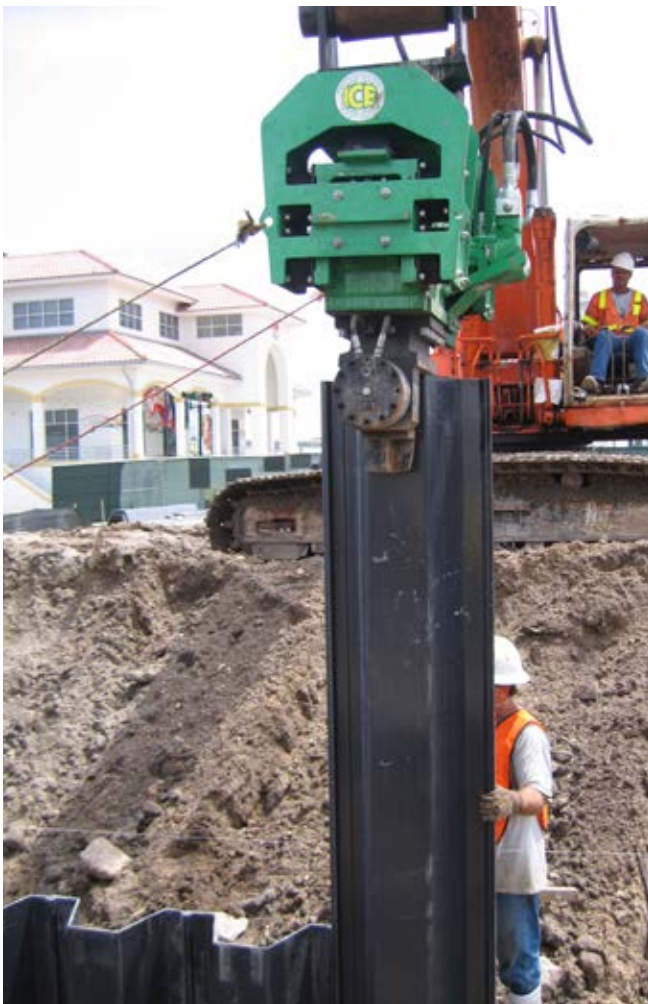
Vibratory Hammer Installation Example
