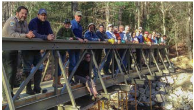
Mtn. Creek Trail Bridge, Pennsylvania
