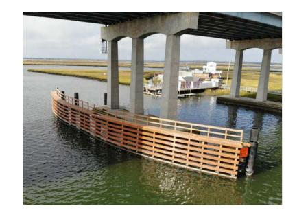
substantially greater energy absorption, deflecting and recovering their shape without damage to the vessel or the fender.
