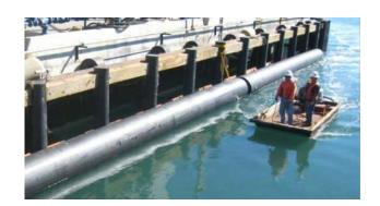
Submarine Camels. Similarly, submarine camels are shaped to facilitate proper spacing between submarines and a pier or wharf. Low maintenance reduces operational costs over traditional steel and wood camels (which require repairs every two years).
